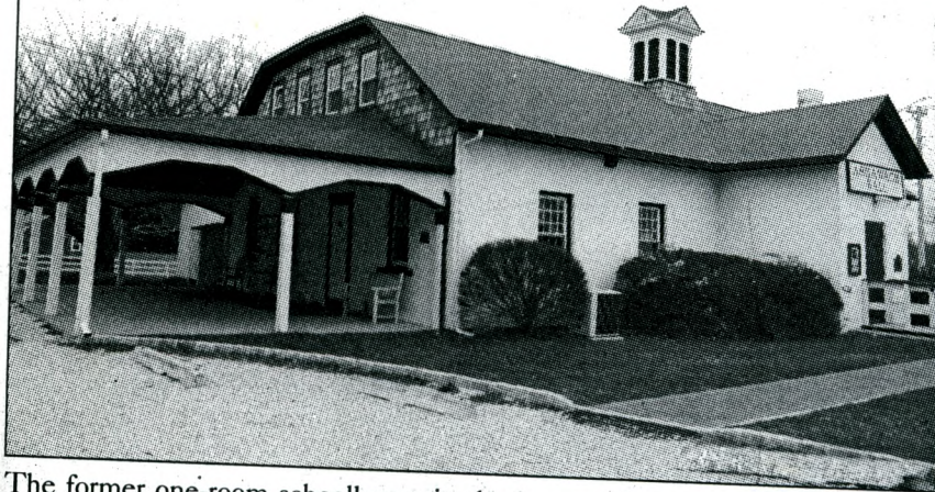
The former one-room schoolhouse in the heart of Springs will have its foundation shored up.
